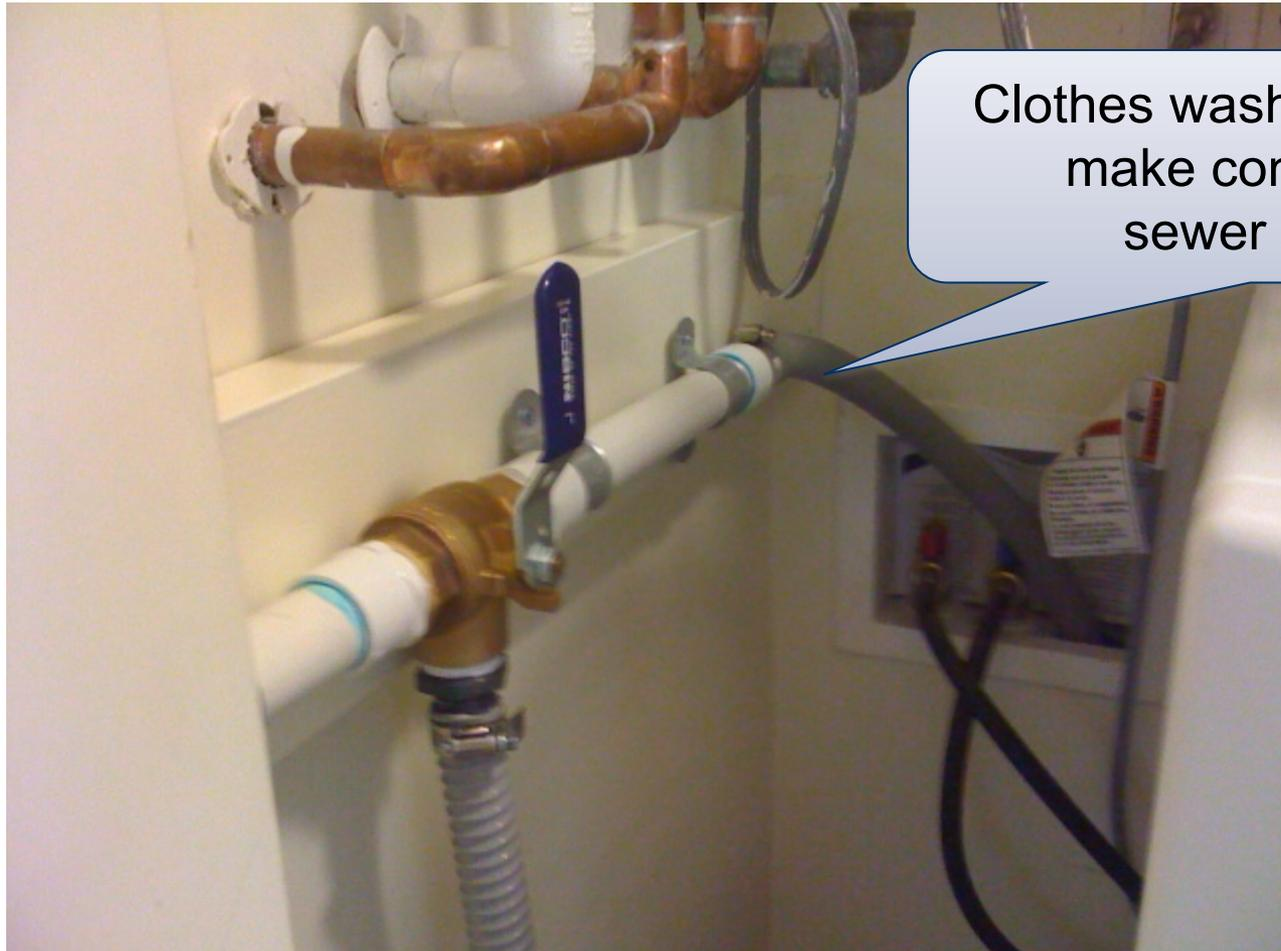
Clothes washer hose used to make connection into sewer standpipe
