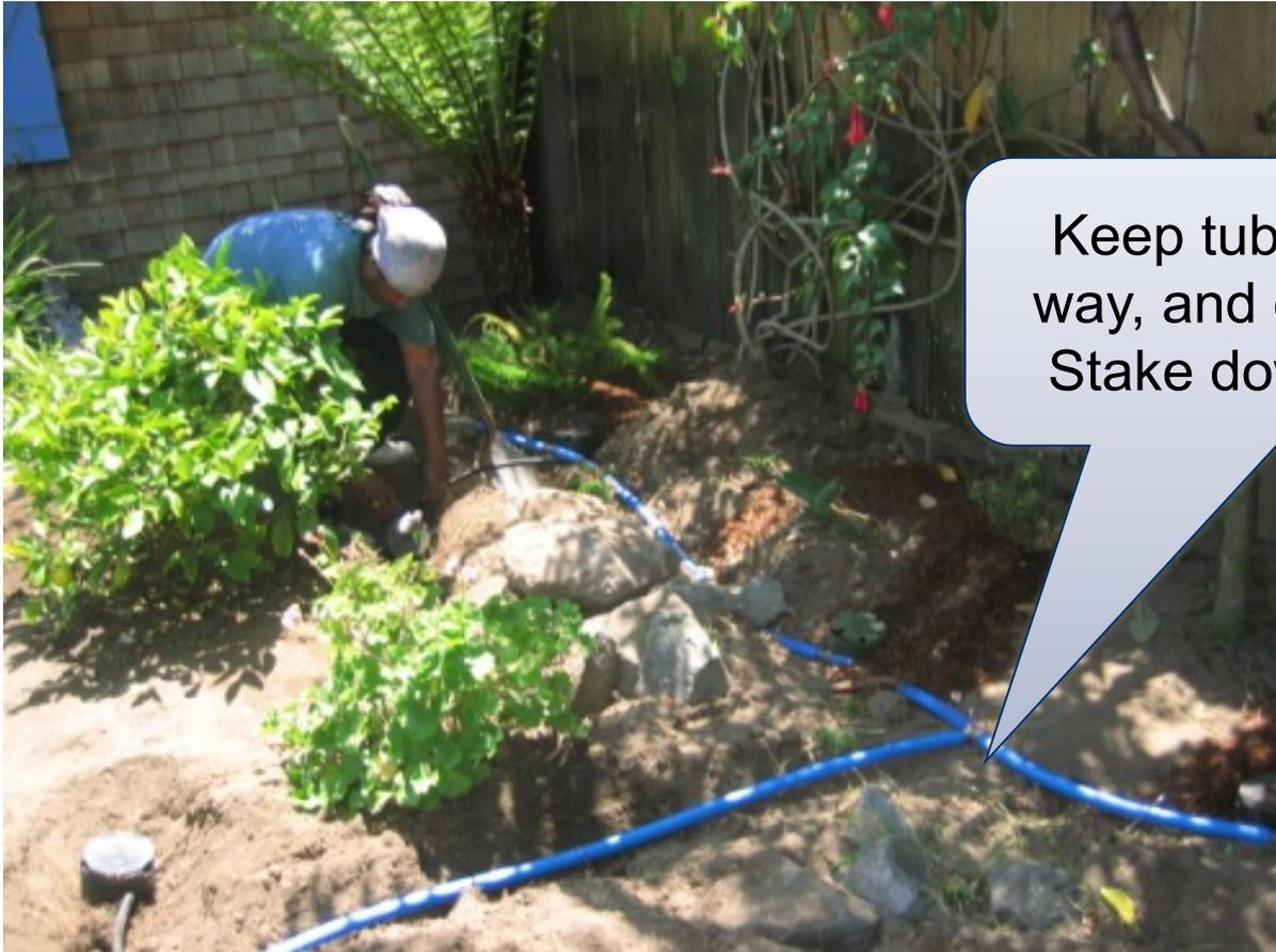
Keep tubing out of the way, and out of sunlight. Stake down as needed
