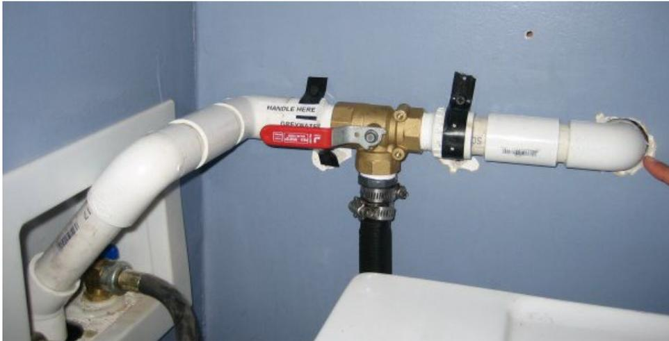
1. 3-way Valve must be above “flood rim” of machine
