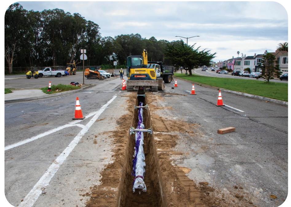
San Francisco Zoo Recycled Water Project: Installation of water pipeline on Sloat Boulevard at Skyline Boulevard.
