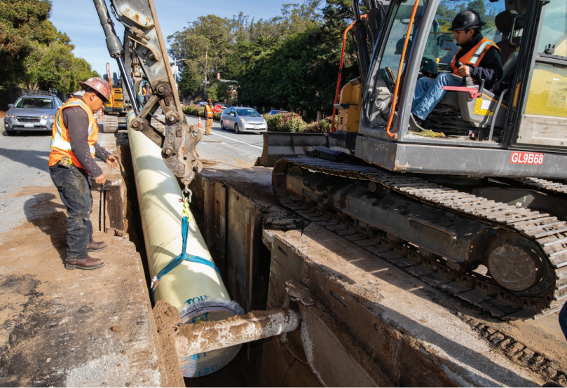
Left: Installing new 36-inch (36") diameter welded steel pipe (WSP) for Potable Emergency Firefighting Water Systems, Right: Harry Tracy Water Treatment Plant (HTWTP), Photos by: Robin Scheswohl
