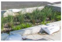
Rain gardens capture stormwater runoff from streets, roofs, and parking lots. Plants and soil absorb that water, reducing the amount of runoff entering the sewer system. This project has constructed a total of 30 rain gardens covering **21,095 square feet of land** between Sloat Boulevard and Irving Street.
