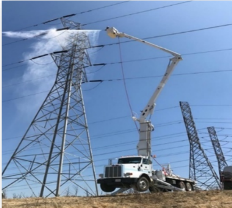
Figure 13 – HHW Line Crew Hot Washing
