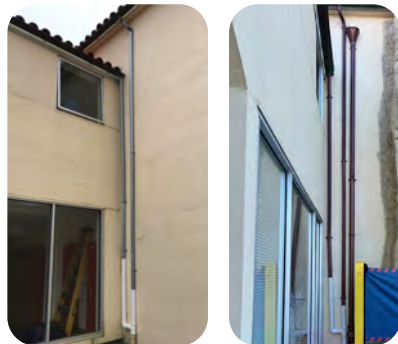
ROOF DRAIN DOWNSPOUT
