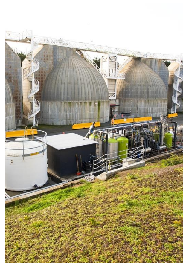
Oceanside Treatment Plant
