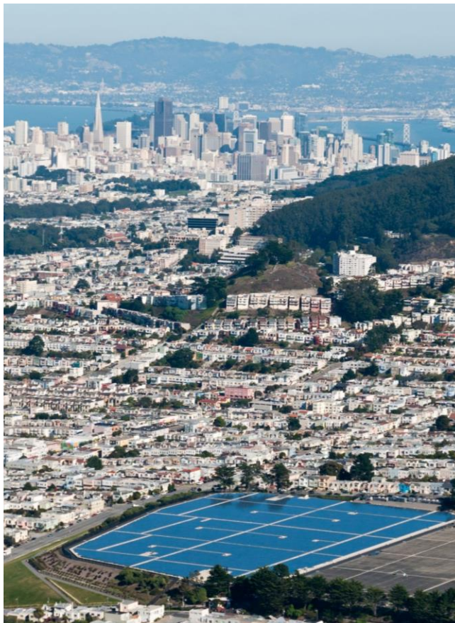
Solar Panels at Sunset Reservoir
