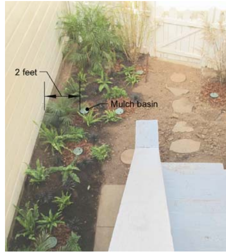
Sample image of a completed graywater system after installation and planting. Photo: Josh Lowe.
