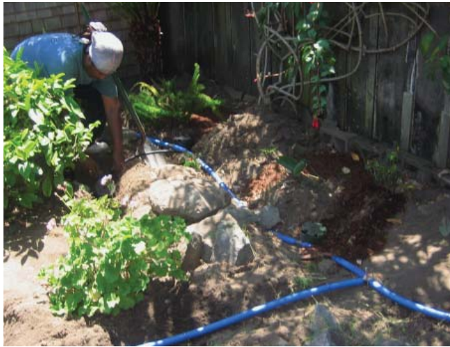
1-inch Blu-lock HDPE tubing laid out in trenches. All tubing is buried after system is installed. Photo: Laura Allen.
