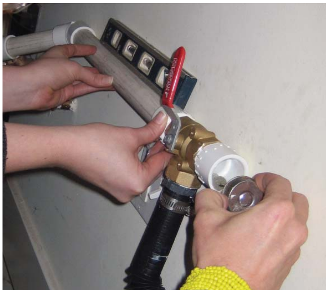
Gluing pipes on either side of a 3-way valve. Photo: Laura Allen.
