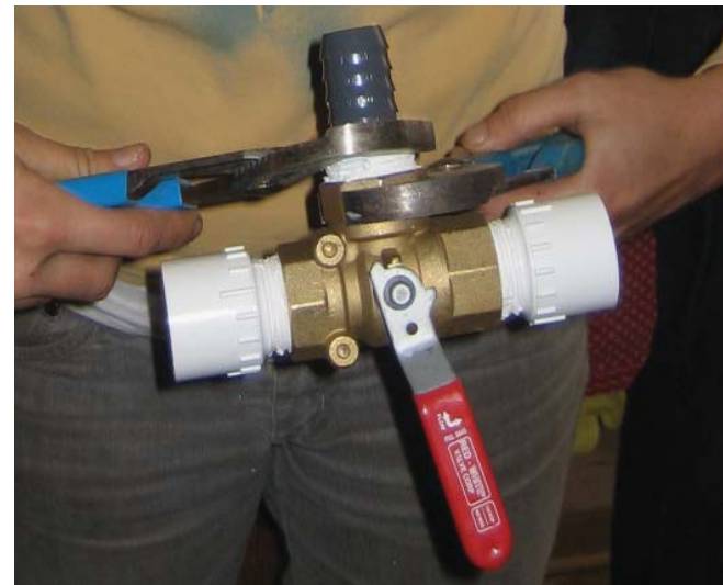
Tightening fittings onto the 3-way valve with channel locks. Photo: Laura Allen.
