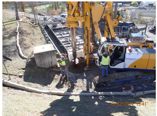
Drilling for Temporary Shoring Adjacent to the Existing Wastewater Treatment Plant
