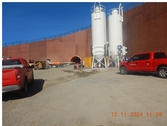
Grout Plant at Priest Adit for Contact Grouting during Outage No. 4
