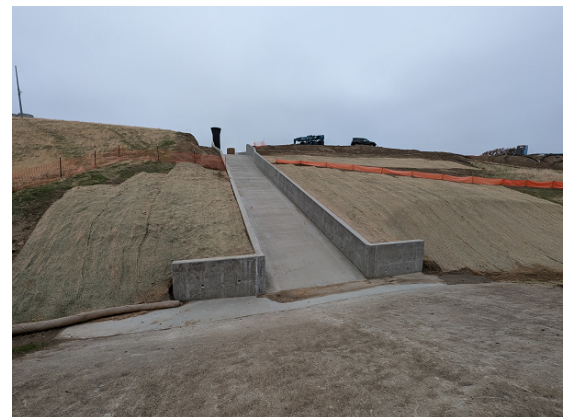
Reinforced Concrete Spillway Rebuilt at Tesla Surge Tower Site
