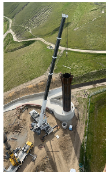
Placing the new Tesla Surge Tower
