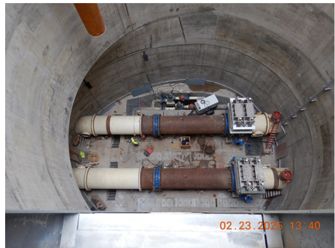
Newly Installed 72 inch Double Disc Knife Gate Valves at Bottom of FCF Shaft
