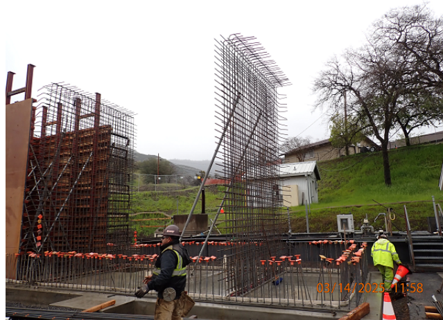
Installation of reinforcement steel for MWWTP walls
