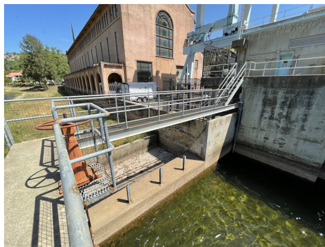
Tie in Location of Bypass to Powerhouse Tailrace
