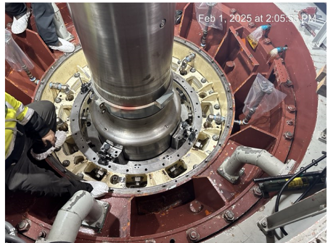
Reading Generator M1 Shaft Runout Measurements
