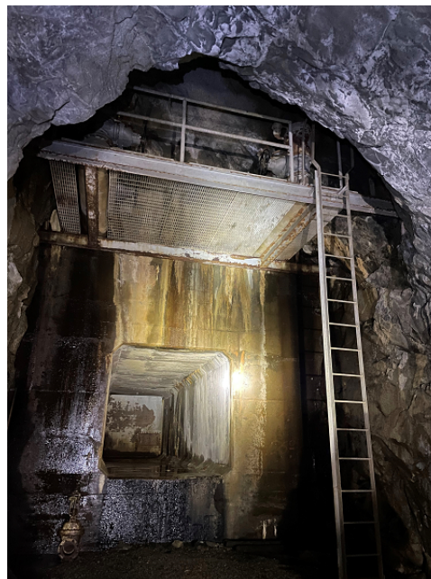
Canyon Tunnel - Hetchy Adit Bulkhead
