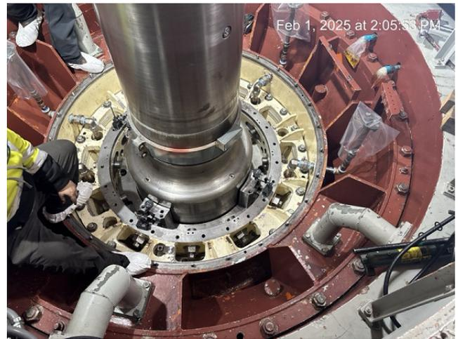
*Measurements of Generator M1 Shaft Alignment*
