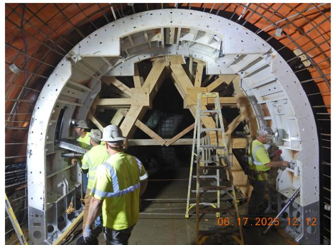
*Installing Forms for the Concrete Lining in the Priest Adit*
