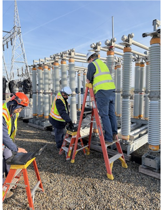
Warnerville Substation: Pretesting City Furnished High Voltage Switches
