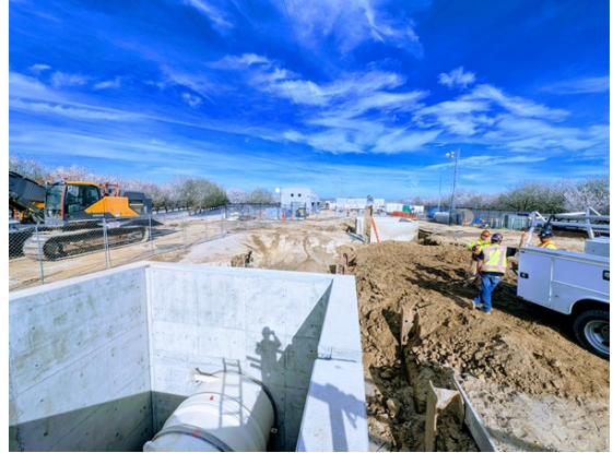
San Joaquin Pipeline Valve and Safe Entry Newly Backfilled Removable Spool Piece Vault at Pelican Valve House, Prior to Lids being Installed
