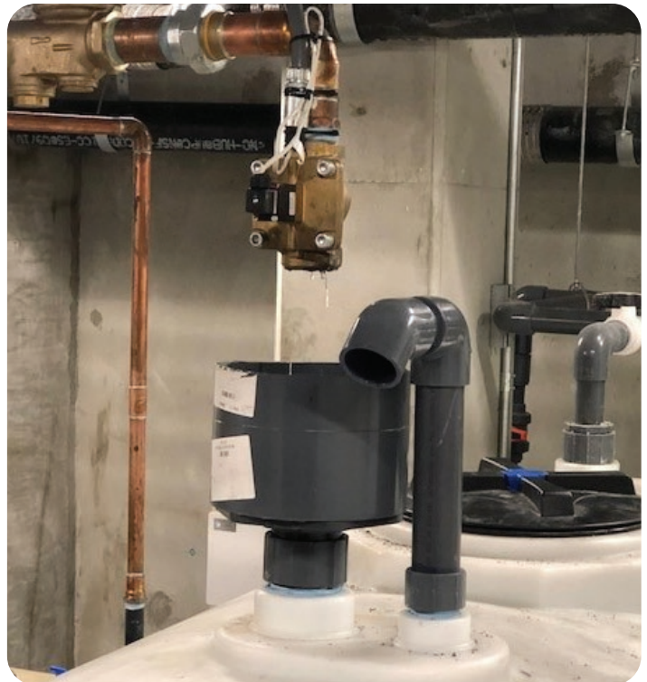
Potable make-up water is supplied to the treated water storage tank via an air gap.
