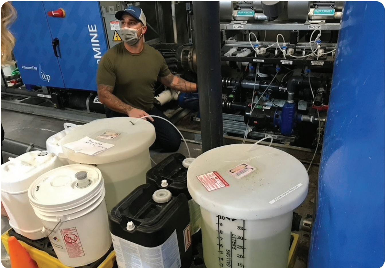
The Treatment System Manager of the combined graywater and rainwater treatment system at 1550 Mission uses chlorine to maintain a disinfectant residual to provide protection against opportunistic pathogens such as Legionella.
