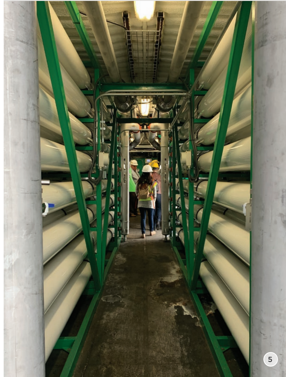
Energy Center San Francisco's closed circuit reverse osmosis system (image courtesy of SFPUC)
