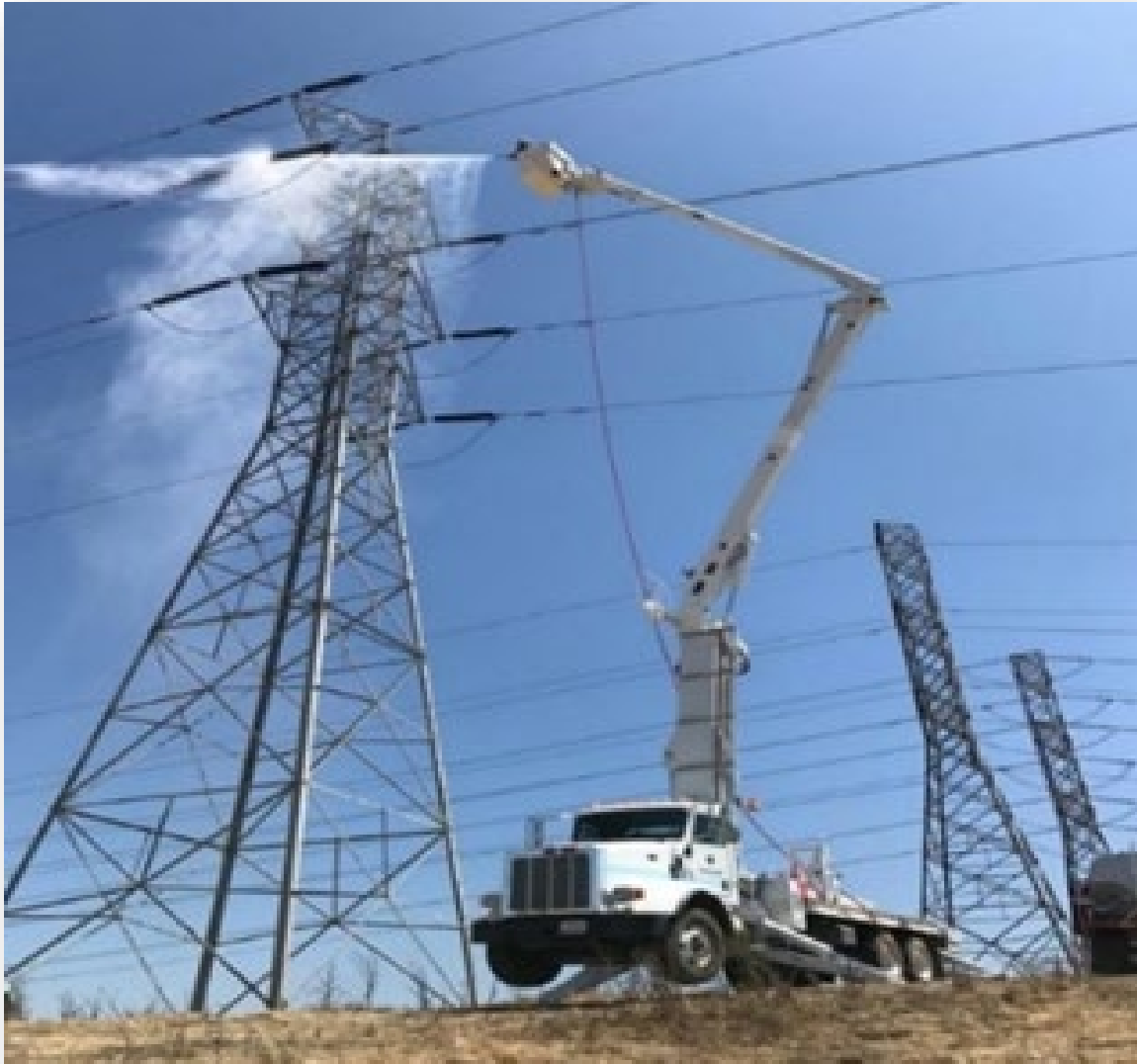
Figure 13 – HHW Line Crew Hot Washing
