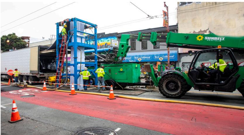
Where possible, we use cure-in-place-pipe (CIPP) to reduce the impact and duration of our work in the street. This method can often reduce the duration of work.
