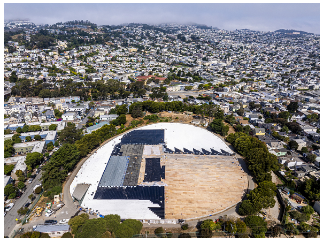
Reservoir Roof Membrane Installation approaching 50% Completion
