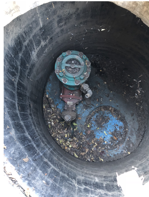
Below-Grade Air Valve to be Upgraded
