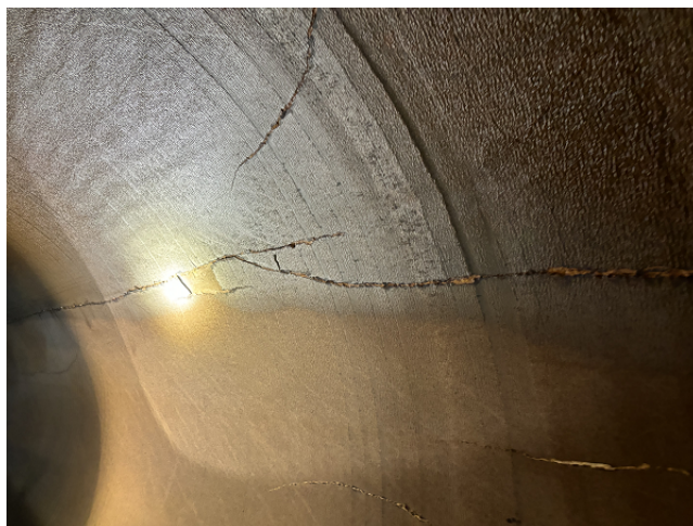
Lining Cracks to be Repaired
