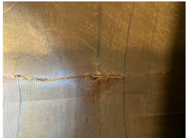
Lining Crack to be Repaired
