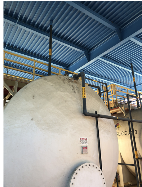
Fluoride Tank at Chloramination Facility
