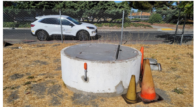
Test Station on Bay Division Pipeline 3 near Stierlin Rd Mountain View
