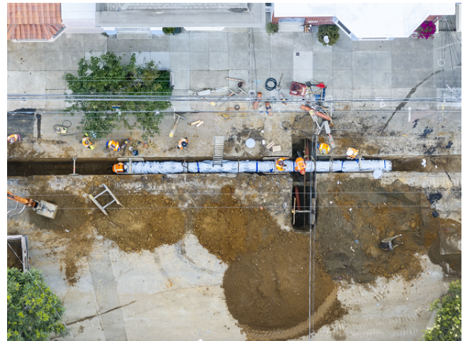
Installation of Earthquake Resistance Ductile Iron Pipe for the Hampshire Street Project
