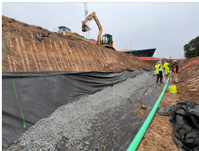
Keyway Excavation and Drainage System
