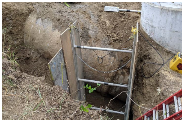
PCCP to Steel Pipe Transition
