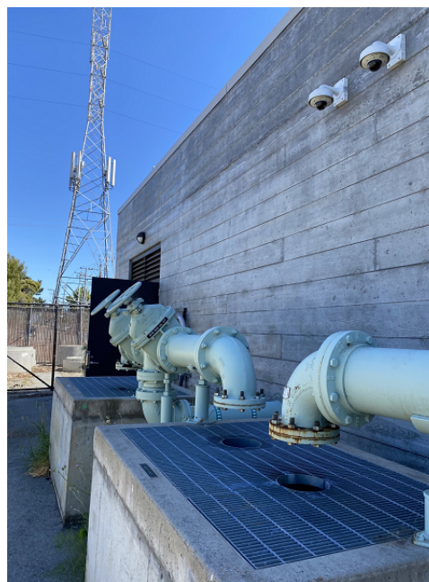
Groundwater Discharge Piping
