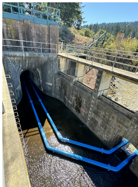
Siphons Installed in Spillway Forebay
