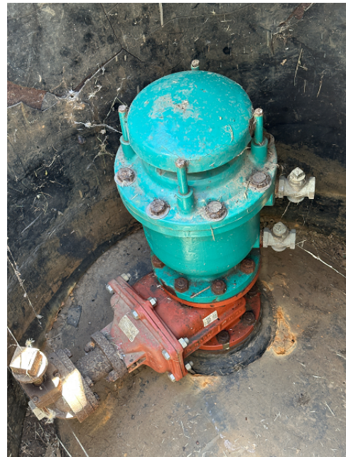
Air Valve to be Upgraded
