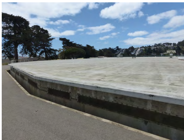
Existing Coating of the University Mound Reservoir
