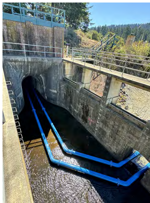
Siphons Installed in Spillway Forebay
