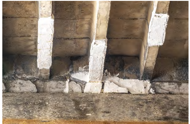
Interior Concrete Spalling
