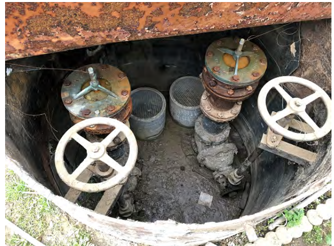
Typical Air Valves to be Upgraded
