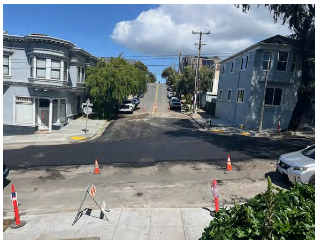
Curb Ramp Construction and Final Paving at Cortland and Prospect
