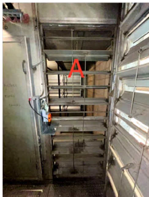
Existing Damper inside the Millbrae Yard Administration Building
