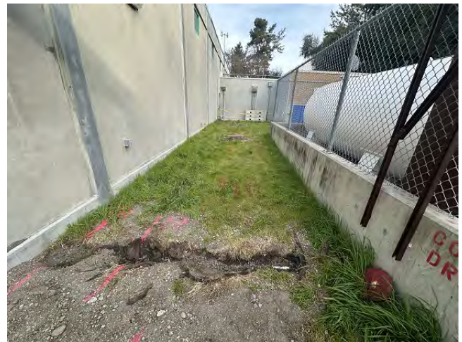
Potholing of Existing Utilities to be Relocated
