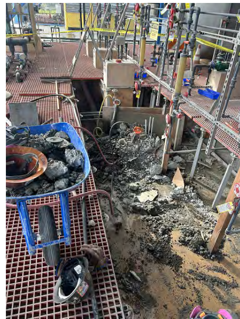
Demolition of Concrete Pump Pedestals
