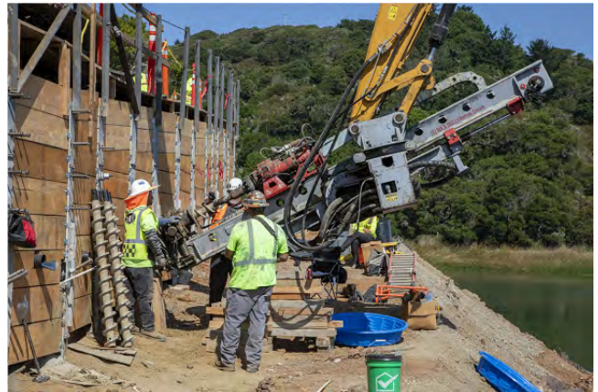
Tie-back Drilling at Ingoing Road
