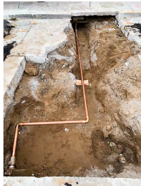
New Copper Piping on Geary Street
