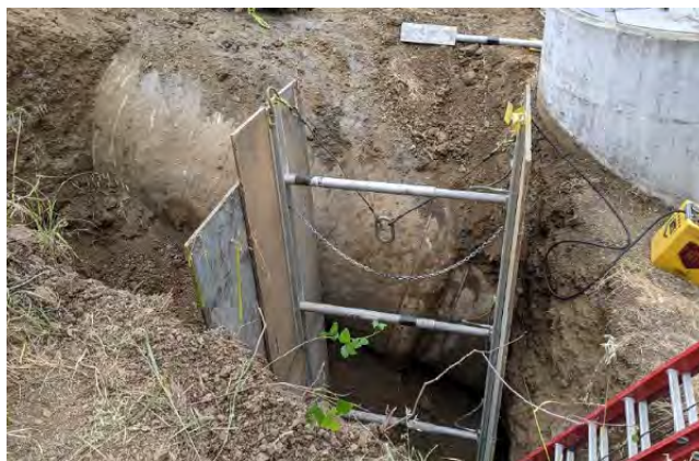
PCCP to Steel Pipe Transition
