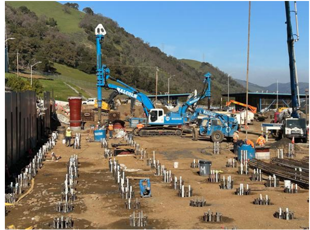
Ozone Contactor Structure Drilled Piers
