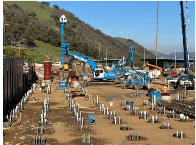
Ozone Contactor Structure Drilled Piers
