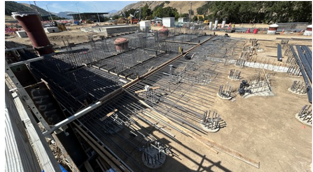
Ozone Contactor Structure Rebar and Conduits
