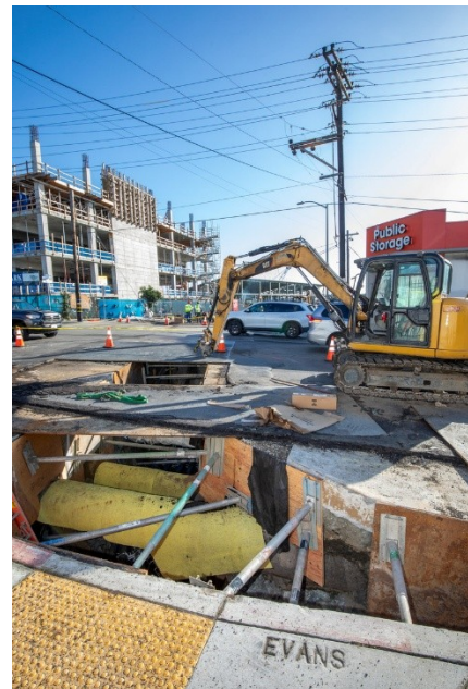
2000 Marin EFWS Pipeline Expansion
