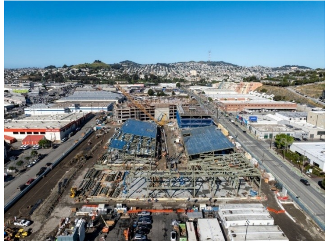
New San Francisco Water Division Headquarters Construction
