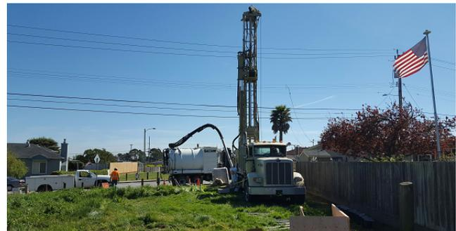
*Typical Anode Well Drilling*
