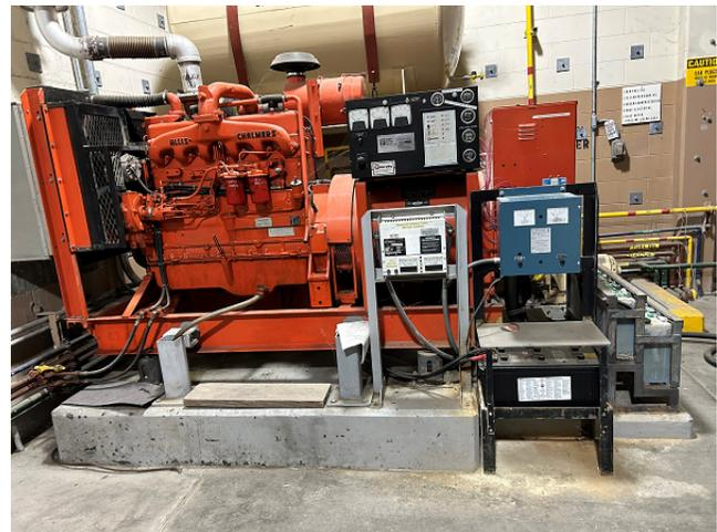
*Existing Diesel Emergency Generator in SAPS Facility to be Replaced with New Propane Generator for Backup Power*
