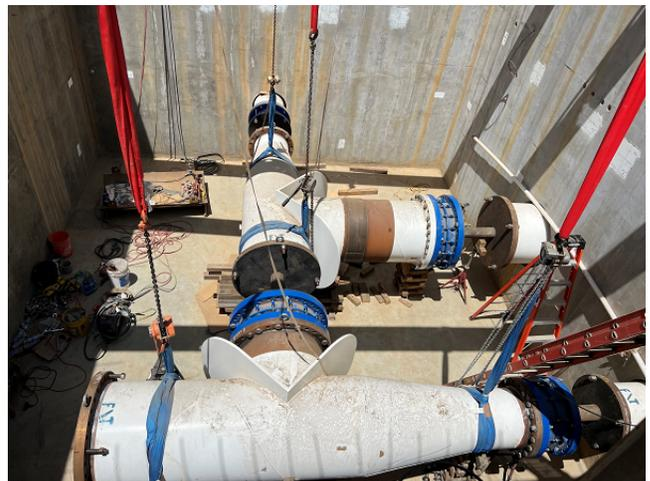
*Inside of Valve Vault with recently installed Valve Manifold Piping*
