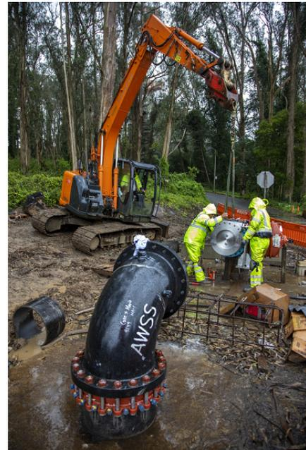
*Installing Valve at the Clarendon Supply Project*
