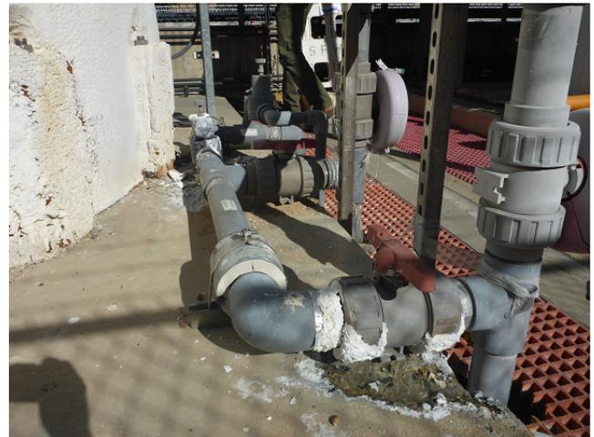
*Concrete Damage at Caustic Soda Line*
