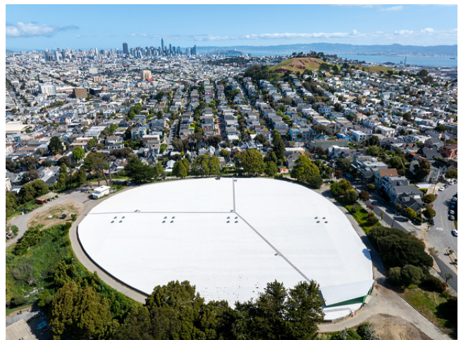
Aerial View of Completed Roof Membrane at College Hill Reservoir
