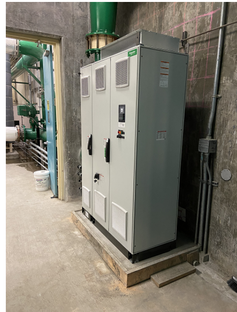
New Variable Frequency Drive for New Air Scour Blower Motor
