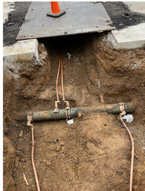
New Copper Piping Water Services on Cityview Way
