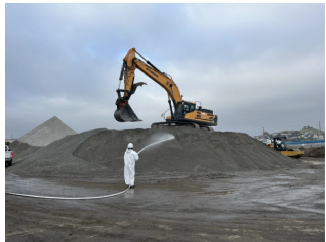
Reuse of Concrete from Existing Building
