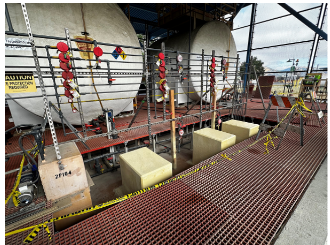
New Coated Concrete Pump Pedestals
