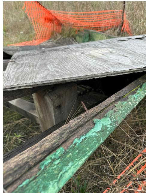
Deteriorating Flexible Joint Coupling Enclosure
