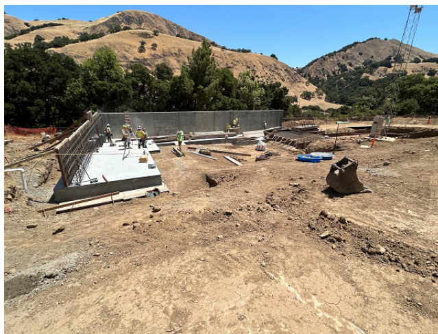
Liquid Oxygen Facility Concrete Retaining Wall
