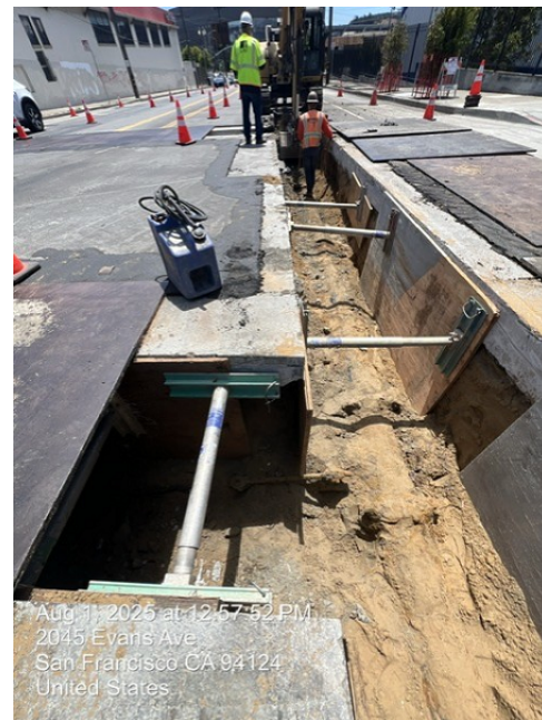
Contractor excavating existing EFWS pipeline expansion connection at the intersection of Evans and Martin
