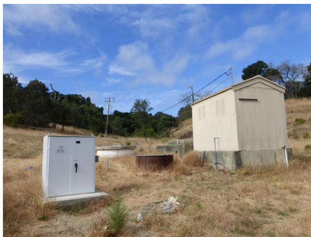
Cathodic Protection Rectifier Installed for the BDPL 3 and 4 Near the Stanford Tunnel Valve House East
