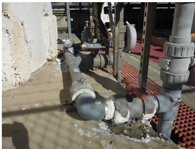
Concrete Damage at Caustic Soda Line
