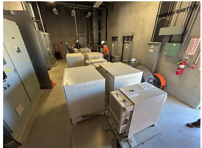
Existing Uninterruptible Power Supply Units
