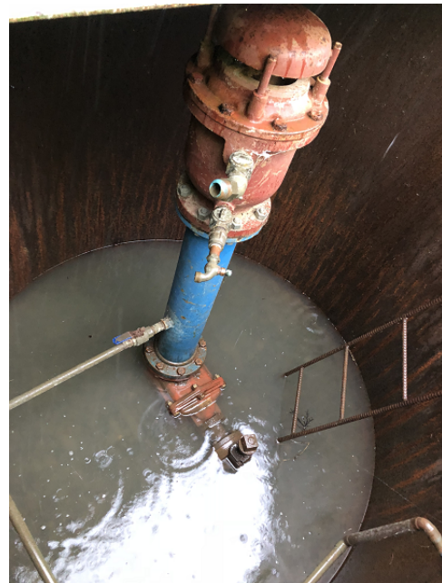
Typical Air Valve to be Upgraded
