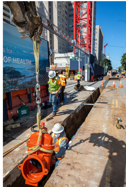
Installing a 12-Inch Ductile Iron Water Pipeline on Parnassus Avenue
