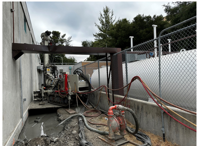
Drilling of Micro-piles for Seismic Upgrades
