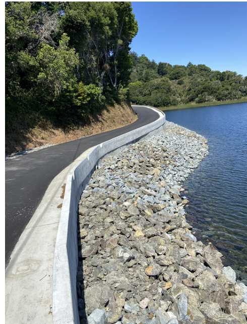
New Soldier Pile Retaining Wall at Ingoing Road Completed in Fall 2024
