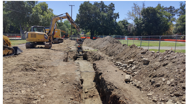
Backfilling New Pipeline Trench
