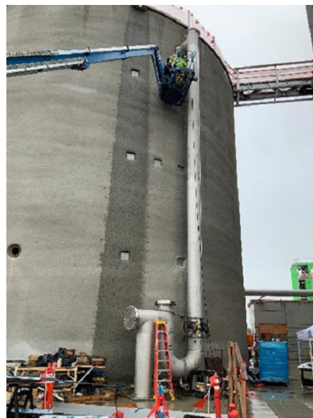
Digester Overflow Piping (Facility 610)
