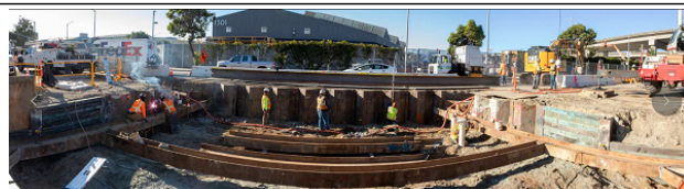
Contract A: Excavation of Vault Area and Installation of Shoring with Bracing
