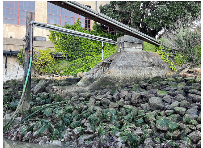
Damaged Rip-Rap Under and Around Laguna CSD
