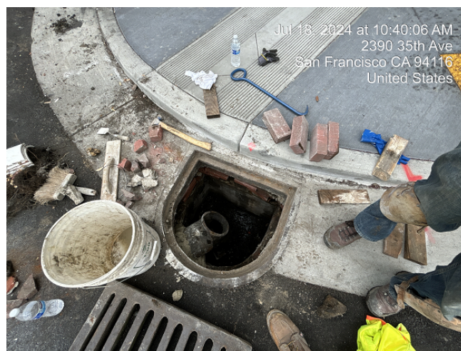
Segment B: Installing Catch Basin Sand Trap and Grouting Joints NE 35th Ave
