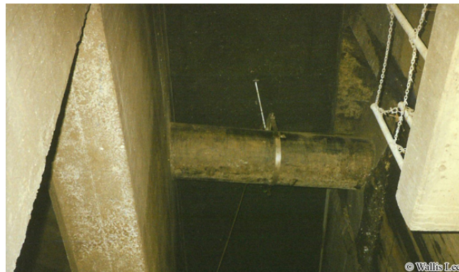
Existing Weir Structure where Marin Street Sewer Crosses over the Islais Creek Transport Storage Box
