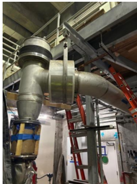
The Contractor continues installation of cogeneration engine exhaust system within Building 800.
