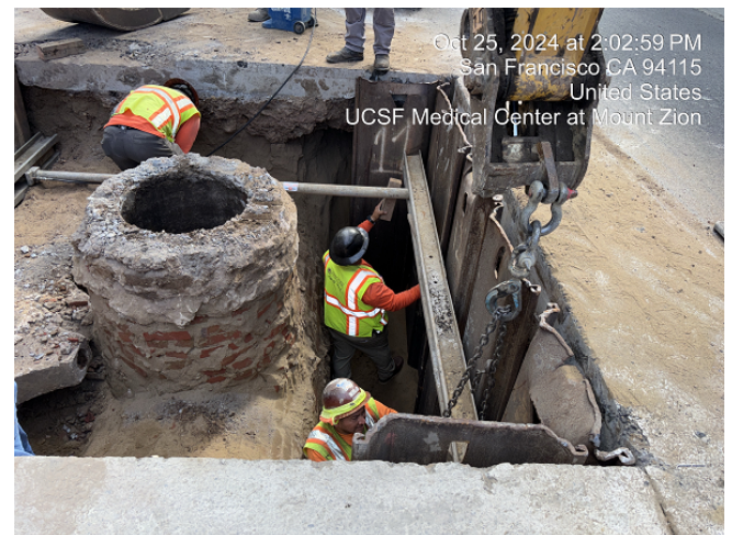
1228I - Shoring for New Manhole at Sutter Street
