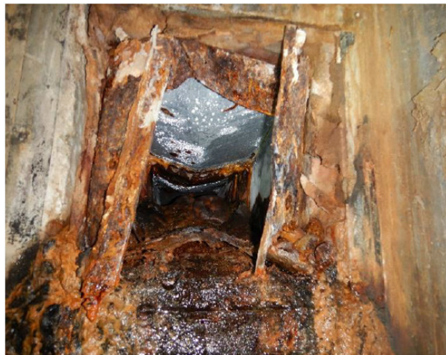
HVAC Ducting Corrosion Due to Water Intrusion
