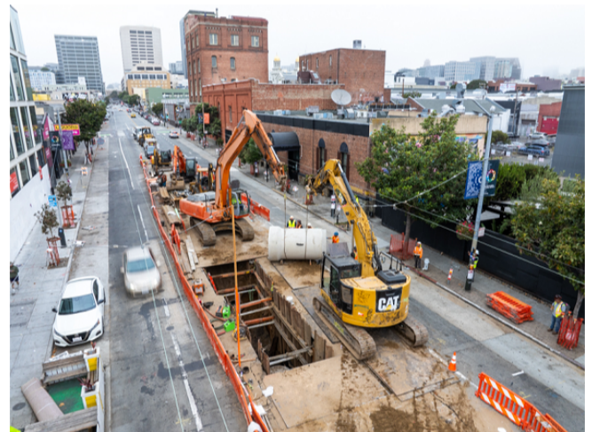
Contract WW-719A installation of 60-inch Reinforced Concrete Pipe on 11th Street
