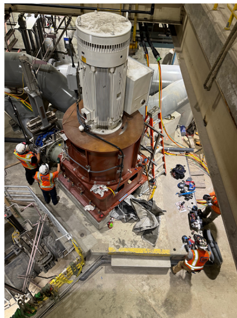
Start-up and Testing of Dry Weather Pump
