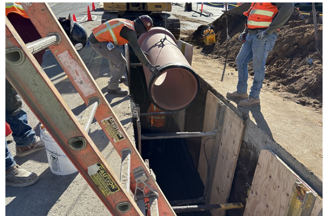
Installation of 24-inch Main Sewer Pipe for Open Excavation Trench on Cordova Street, San Francisco
