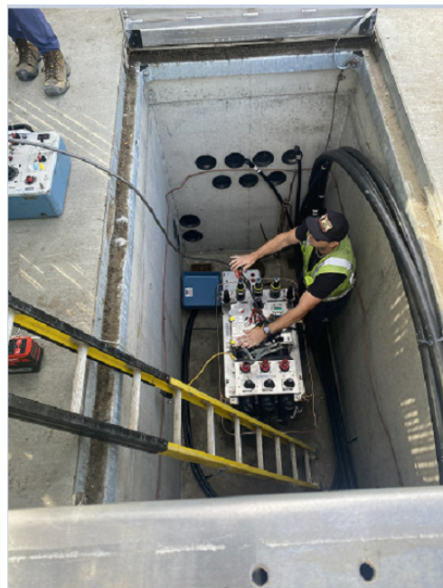
Power Enterprise tested the new interrupter switch assembly and PG&E subsequently energized new primary power service to New Electrical Building
