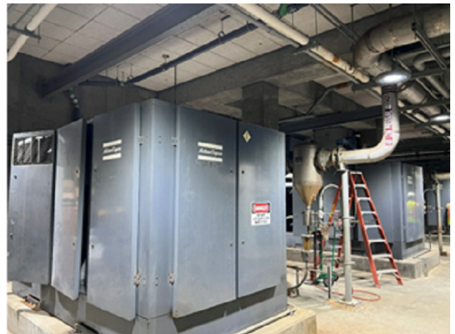
Building 011 existing Pressure Swing Absorption type compressor assembly identified for replacement
