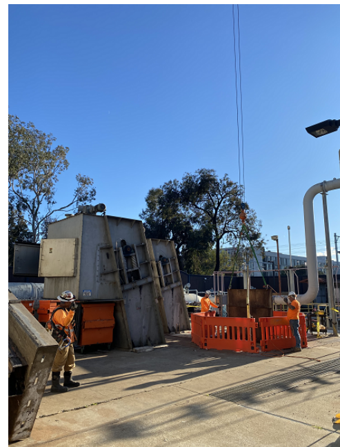
WW-749 Contractor utilizing crane equipment to support demolition of the Channel Pump Station South Channel bar screen assemblies
