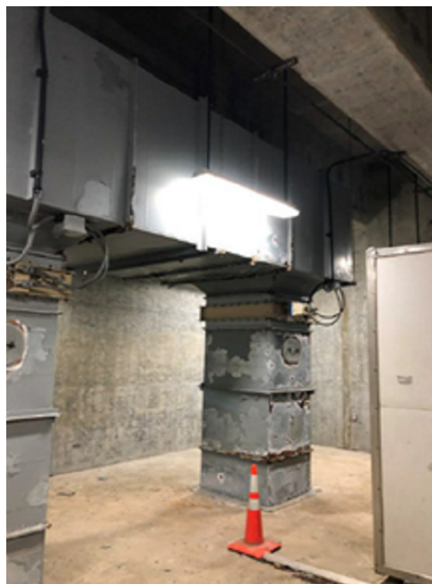
Building 200 corroded ductwork manifold identified for replacement
