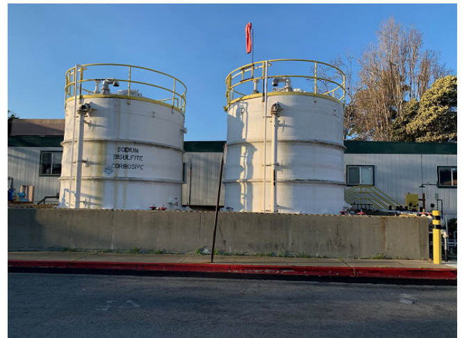
Existing Sodium Bisulfite Tanks
