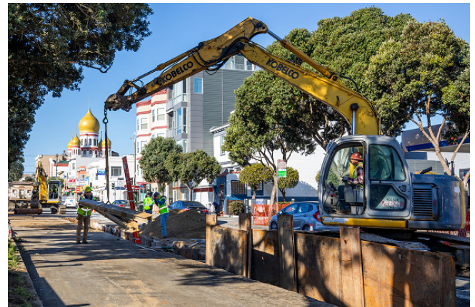
Sewer Installation on Geary Boulevard
