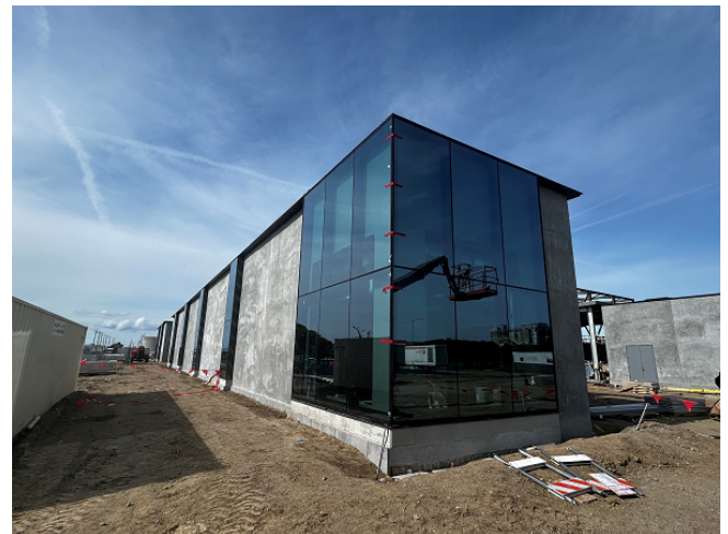
View of the Administration Building Glazing Installation
