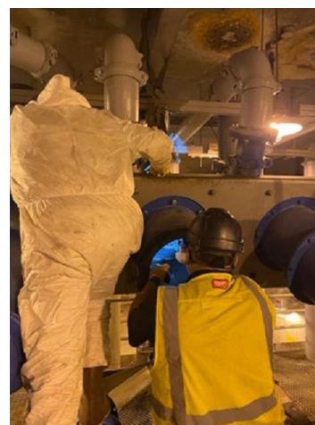
Contract (F) WW-669 Contract work at hydro gritter assembly. Cyclone liner material inspection.
