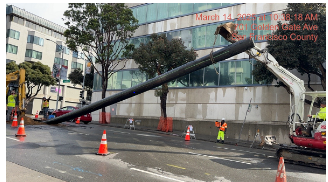
1308R/2815J - Sliplining at Franklin St and Golden Gate Ave Intersection
