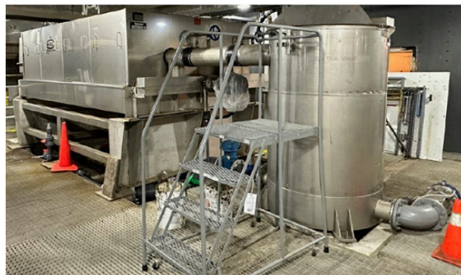
Install two (2) additional Rotary Drum Thickeners assemblies, in positions No. 2 and No. 3, similar to the unit above installed in position No. 1
