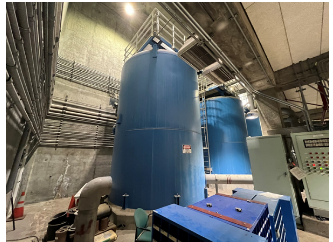
Replace existing Pressure Swing Absorption (PSA) vessels that are at the end of their useful life
