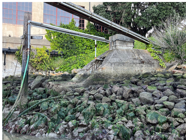
Damaged Rip-Rap Under and Around Laguna CSD
