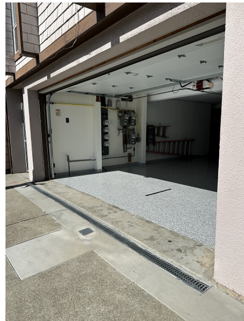
Completed Floodwater Grant Project at 1676 Union St. The Project Included a Trench Drain Across the Garage and Wet Floodproofing to Protect Against Overland Flows
