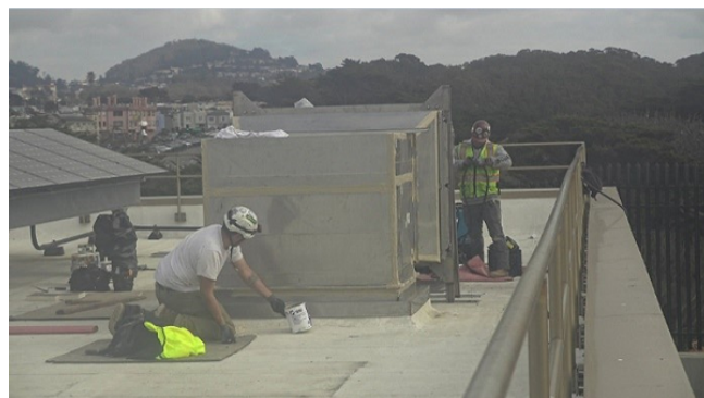
Contractor performing roof top air handler installation work at New Electrical Building.
