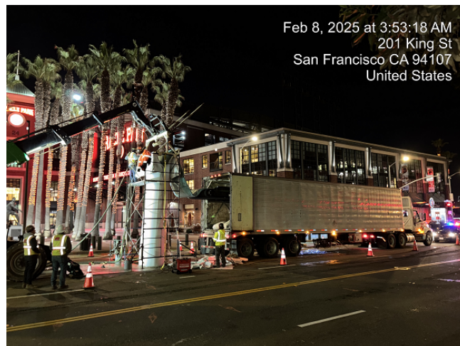
Contract A: Cured-In-Place-Pipe Installation at Night
