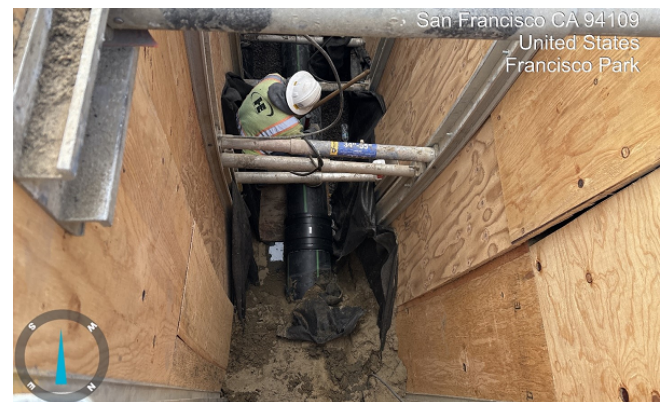
Joining 14-inch Diameter High Density Polyethylene Pipe (HDPE) by Electro-Fusion Welding in an Open Excavation Trench on Bay St
