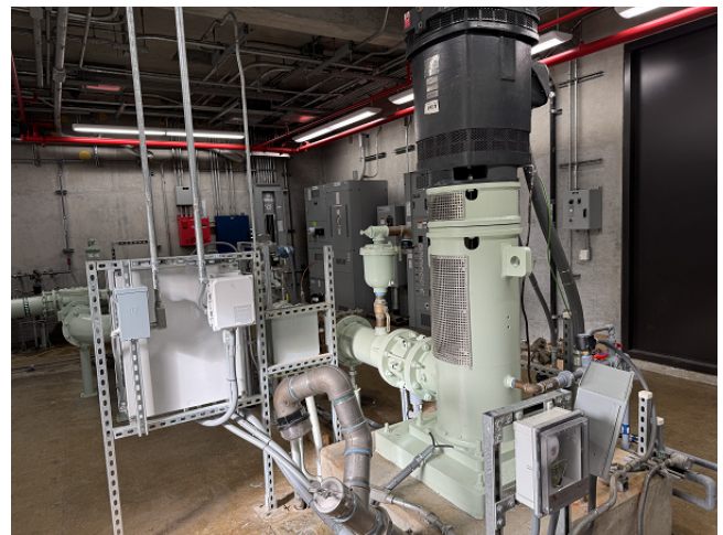
Colma BART - Completed Pump Reinstallation
