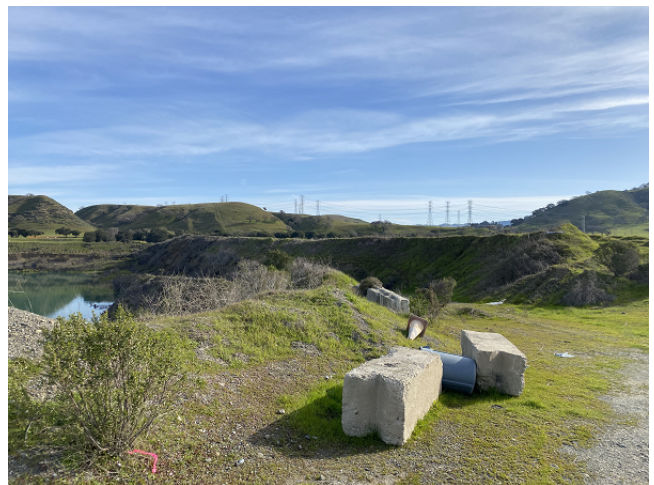
Access Road leading into Pond F2
