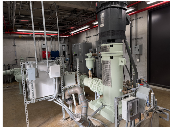
Colma BART - Completed Pump Reinstallation
