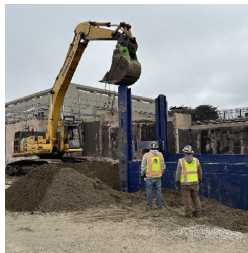
Buried 42-inch Pipe Shoring and Excavation Work on Site
