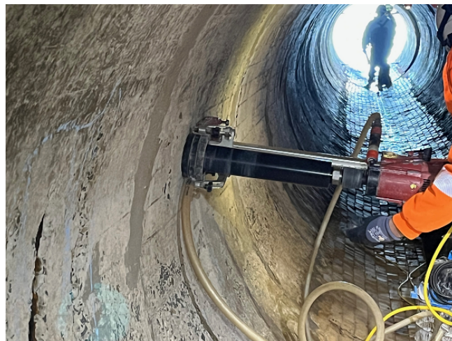
Coring Test at Laguna CSD
