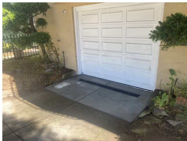
425 West Portal Ave with Newly Installed Trench Drain to Protect the Property Against Flooding from the Public Right-of-Way
