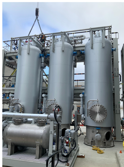
Thermal Hydrolysis Process (Cambi Vessel)
