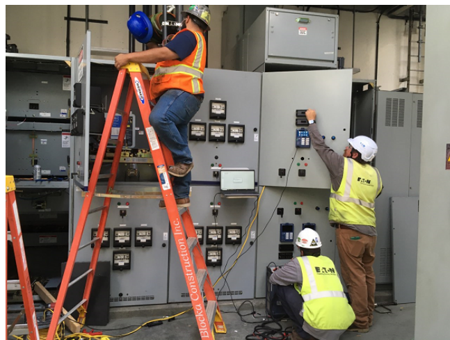
Switchgear Modification at Booster Station
