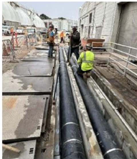
Contractor Installing Pipe Labeling in Utility Pipe Trench
