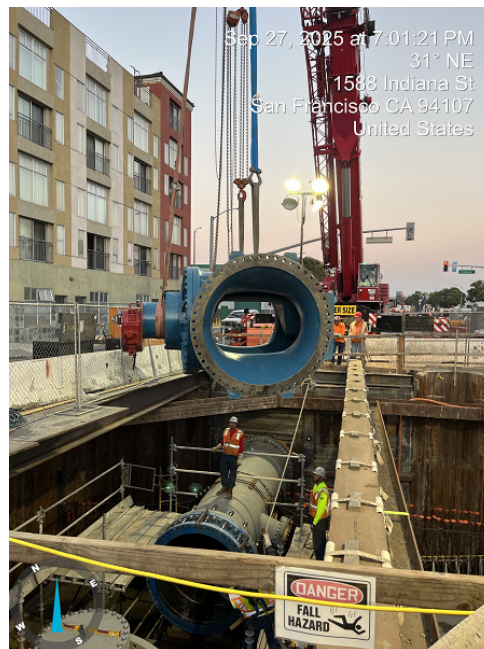
Contract A: Crane Lowering the 66" Plug Valve into Place
