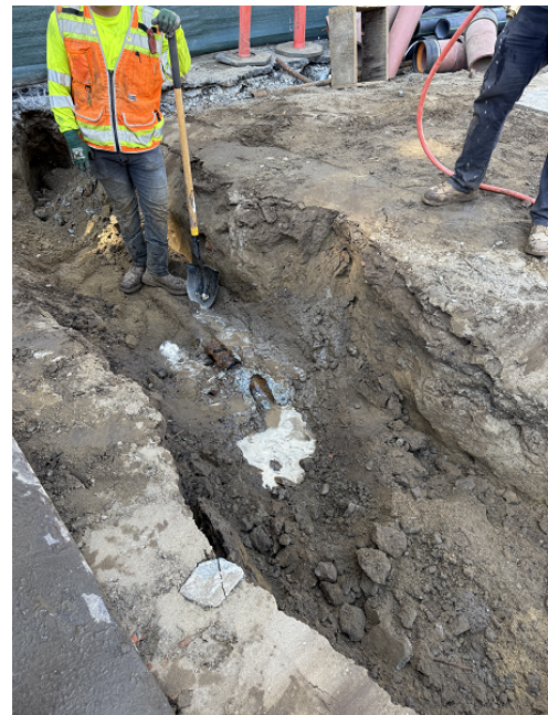
Sewer Lateral Excavation
