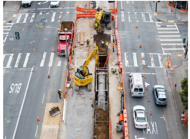
Installation of 42 Inch Diameter RCP on Geary Boulevard at 7th Avenue Under Contract WW-743
