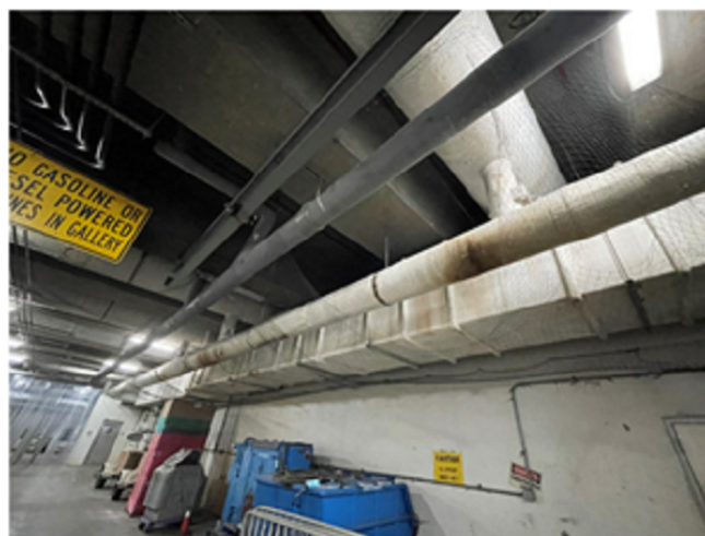
Existing Deteriorated Exhaust Fiberglass Reinforced Plastic (FRP) Ductwork and Associated Duct Supports Serving Building 042 Identified for Replacement
