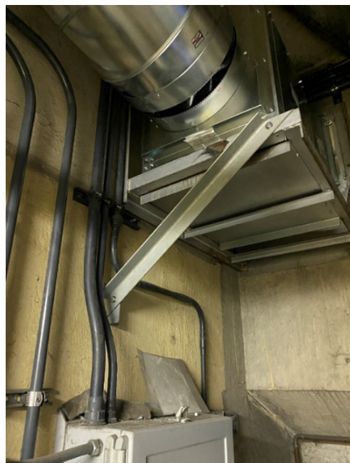
Exhaust Fan Duct Modification
