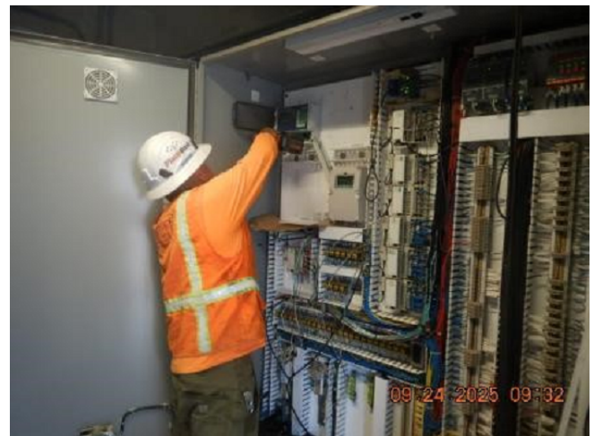
WW-749 Level Sensor Controller Install
