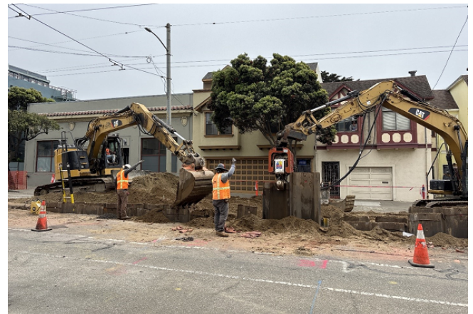
Two Operators Concurrently Working Under De-Energized Muni Overhead Contact System Wires to Efficiently Install 12-inch Diameter Vitrified Clay Pipe and Backfill the Trench on Cabrillo Street, San Francisco
