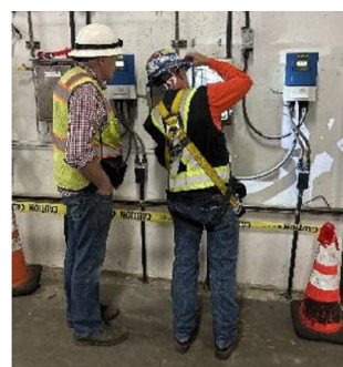
Contract (F) WW-669 Contractor Is Reviewing Performance of 24-inch Influent Butterfly Valve Local Controller During 7-Day Commission Testing
