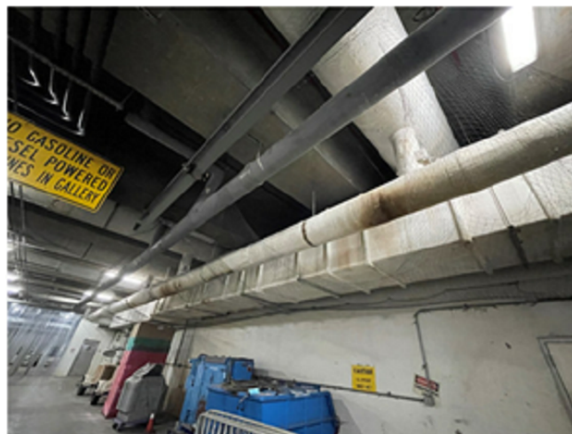
Existing Deteriorated Exhaust Fiberglass Reinforced Plastic (FRP) Ductwork and Associated Duct Supports Serving Building 042 Identified for Replacement
