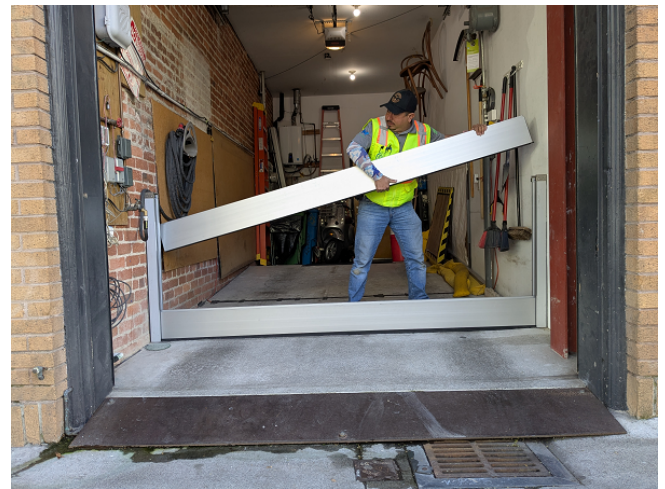
Flood Barrier Being Installed at 2779 16th St.
