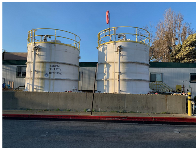
Existing Sodium Bisulfite Tanks
