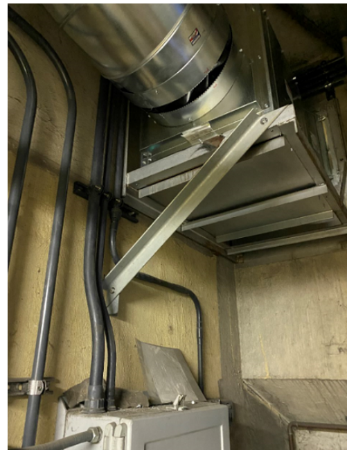
Exhaust Fan Duct Modification
