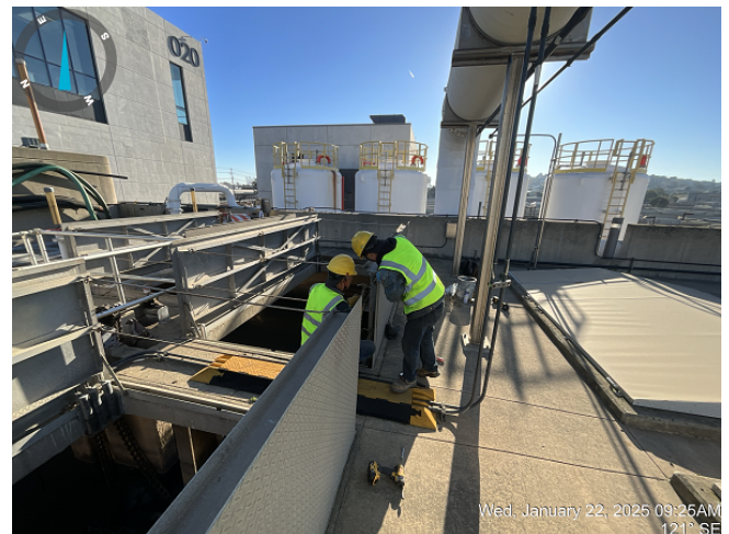
WW-749 Channel Pump Station (CHS). South Channel Cofferdam Install to Support Future Lift Pump Suction Pipe Repairs
