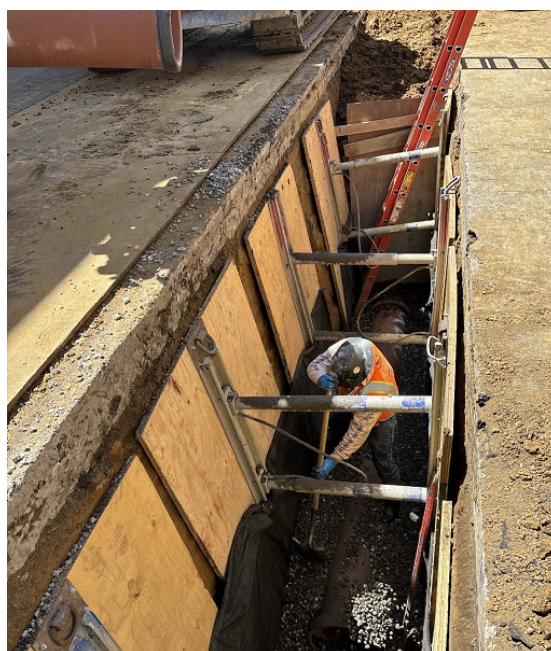
Placing Crushed Rock Bedding Around Newly Installed 12-inch Diameter Vitrified Clay Pipe Using the Shovel Slice Method in an Open Excavation Trench on Pixley Street
