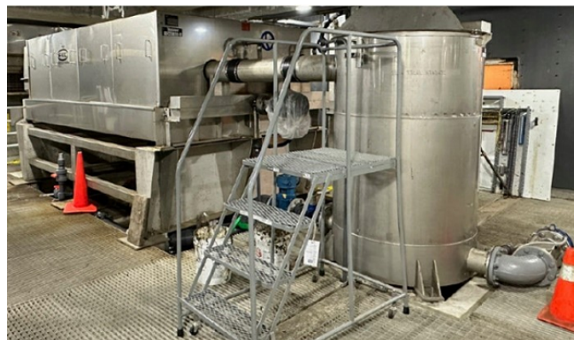
Representative Rotary Drum Thickeners
