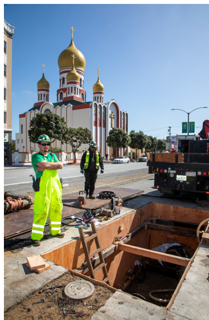
Water Line Connection Pit on Geary Boulevard Under Contract WW-743
