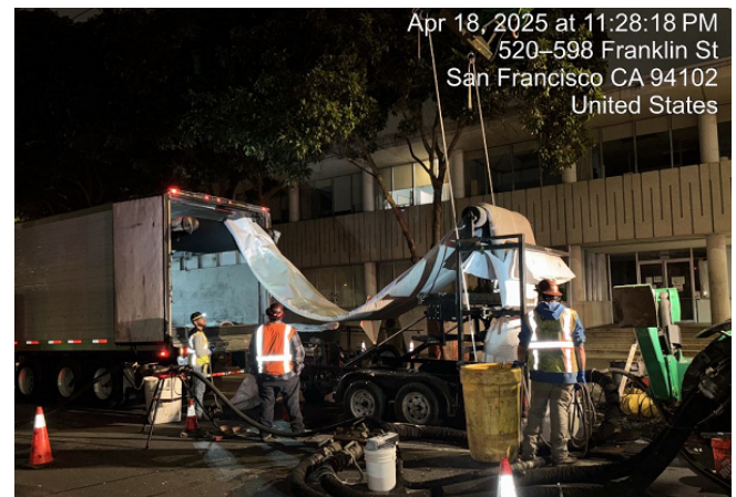
WW-753 Liner Installation at Frankling Street
