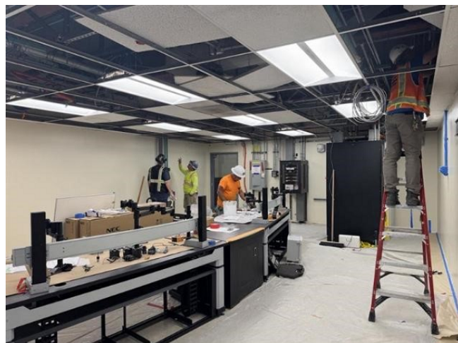
NSS Control Room New Workstation
