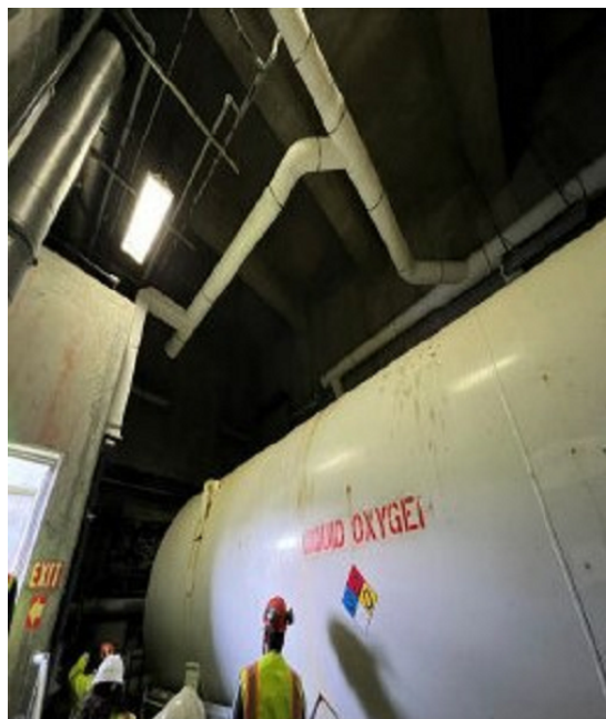
Existing Liquid Oxygen Storage Tank Identified for Replacement
