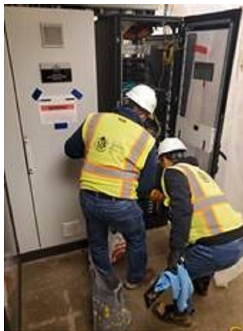
DCS Server Cabinet Maintenance at Northshore Pump Station
