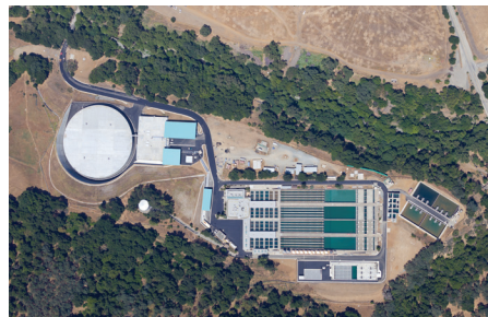
SVWTP aerial view
