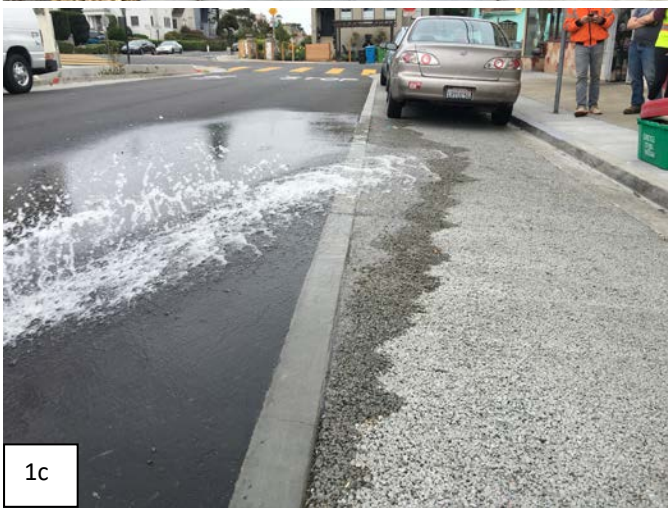
Figure 1a, 1b and 1c: A mid-block sidewalk planter, end-of-block bulbout planter, and pervious concrete.
