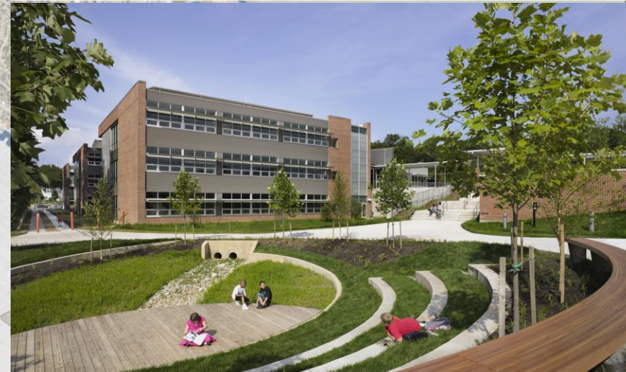
Multi-Purpose Surface Detention / Manassas Park, VA
