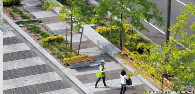
Floodwall with seating Longsdale Street Danenong, Australia
