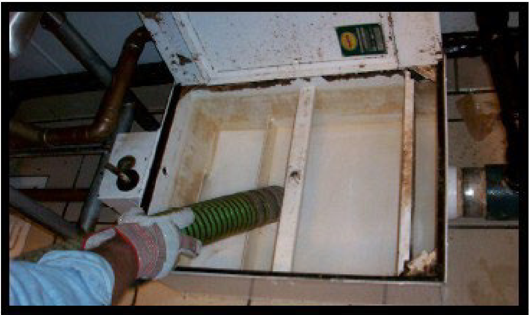
Figure 5. Example of a trap being cleaned by a contractor. Source: Bay Area Pollution Prevention Group
