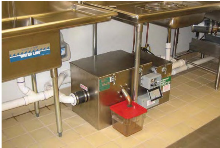
Figure 4. Example of an installed automatic grease removal device. Source: The Wastewater Solutions Update
