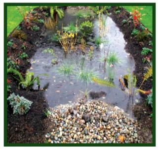
A rain garden experiencing ponding during a rain event. In a functioning rain garden, this ponding should infiltrate into the ground within 24-48 hours. Source: 12000 Rain Gardens
