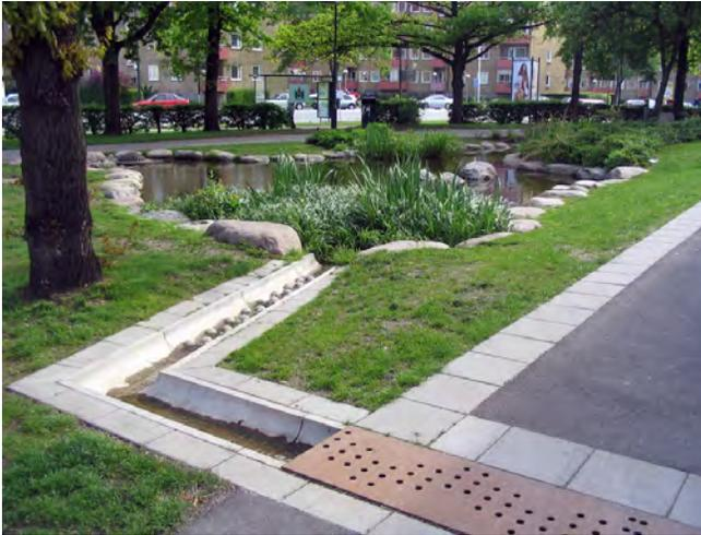
*Conveyance features, such as this trench drain and runnel, can be used to move stormwater between treatment controls.
