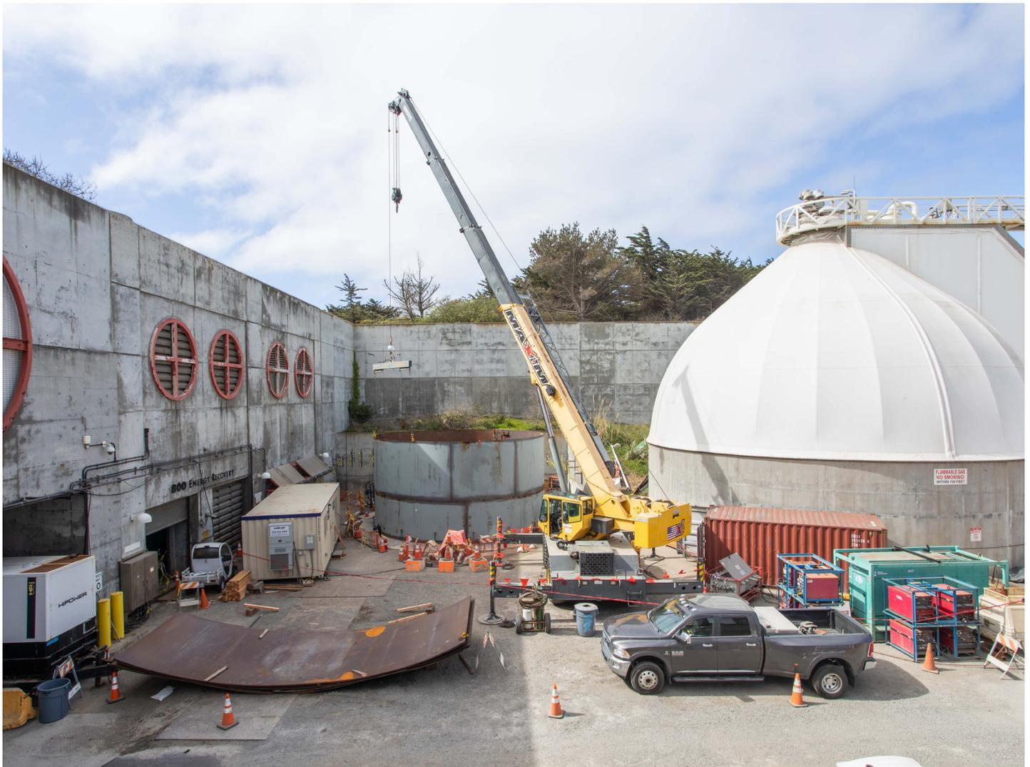
*Oceanside Treatment Plant (OSP) Digester Gas Utilization Upgrade: Fabricating gas holder tank (Building 741) by placing and welding steel plates. Tank will be 59' tall and hold excess digester gas.*
