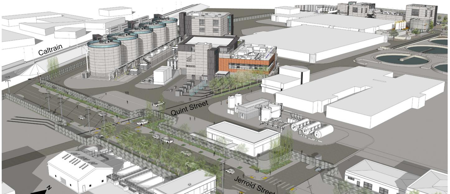
*Rendering of new southeast treatment facilities and relocation of biosolids digesters.*
