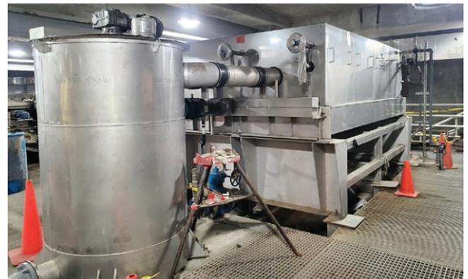
*Proposed New Rotary Drum Thickener (RDT) and Associated Flocculation Tank Assembly*
