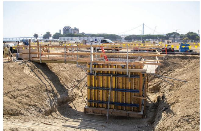
*Installing Formwork for Concrete Placement of Influent Pumping Structure Walls*
