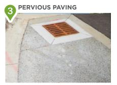
Permeable paving allows stormwater to soak into the ground in contrast to hard surfaces (concrete or asphalt) where stormwater rapidly flows into the sewer system. This project includes 5,475 square feet of pervious concrete to help divert stormwater.
