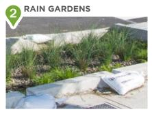
Rain gardens capture stormwater runoff from streets, roofs, and parking lots. Plants and soil absorb that water, reducing the amount of runoff entering the sewer system. This project has constructed a total of 32 rain gardens covering 6,746 square feet between Lands End Trail Eagle Point and the California Coastal Trail entrance at 25th Ave North.
