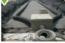
An underground stormwater storage structure filled with gravel that receives runoff through horizontal pipes below the pavement surface. This project includes over 10,347 square feet of infiltration gallery to helps store stormwater and slowly release it into the groundwater aquifer.
