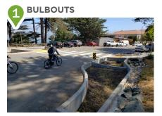
A traffic calming method that extends the sidewalk, reducing the distance to cross the street. increasing pedestrian visibility and safety. These also include green technologies and rain gardens to capture and treat stormwater.
