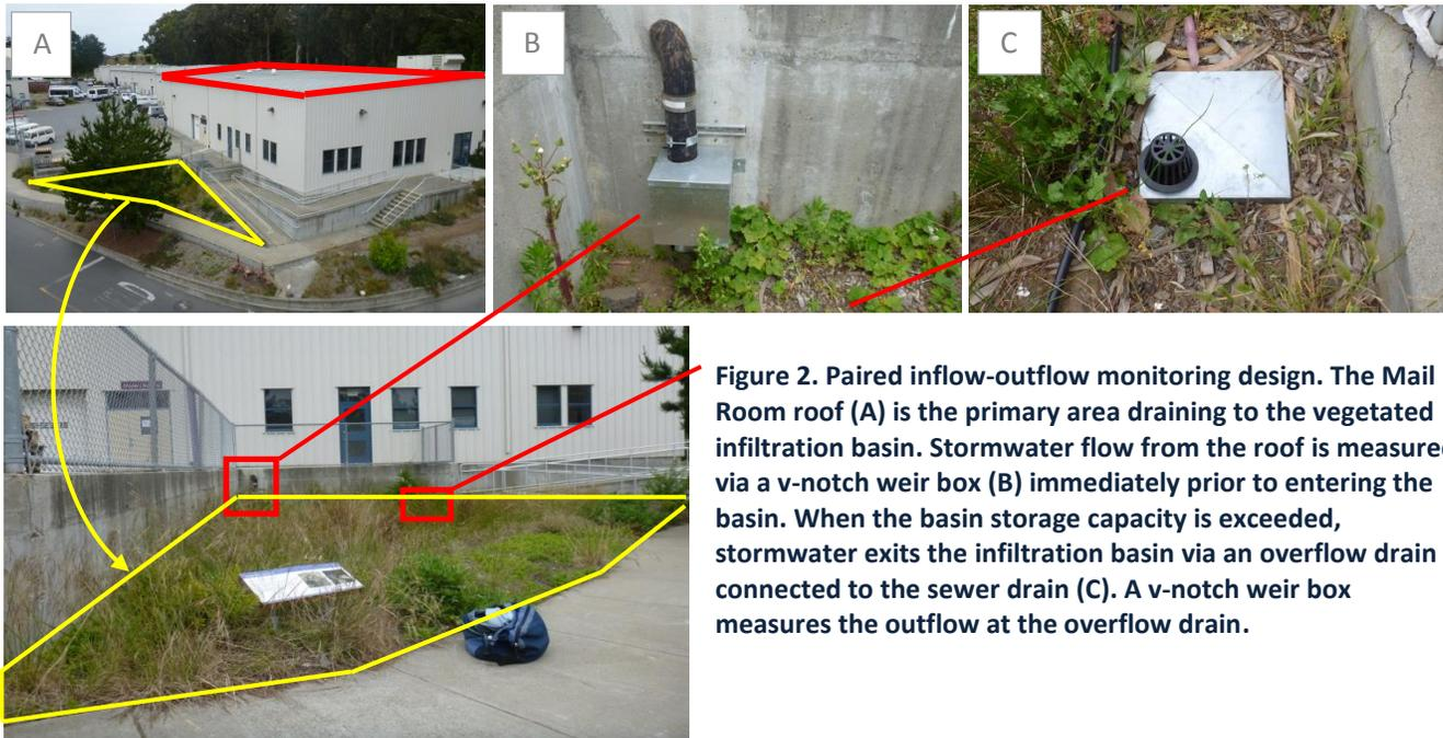
Figure 2. Paired inflow-outflow monitoring design. The Mail Room roof (A) is the primary area draining to the vegetated infiltration basin. Stormwater flow from the roof is measured via a v-notch weir box (B) immediately prior to entering the basin. When the basin storage capacity is exceeded, stormwater exits the infiltration basin via an overflow drain connected to the sewer drain (C). A v-notch weir box measures the outflow at the overflow drain.
