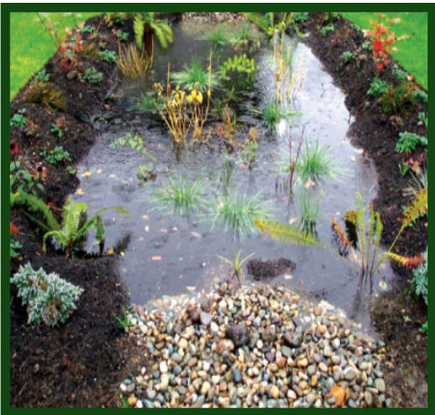
*A rain garden experiencing ponding during a rain event. In a functioning rain garden, this ponding should infiltrate into the ground within 24-48 hours.
